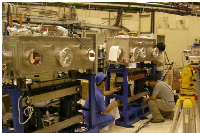
Mirror systems being installed at NSRRC, Taiwan
